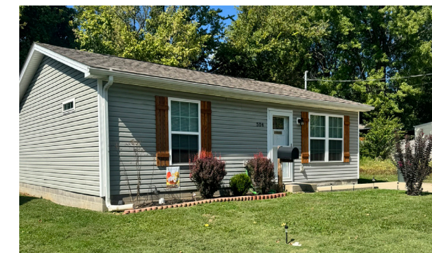
Existing housing example
